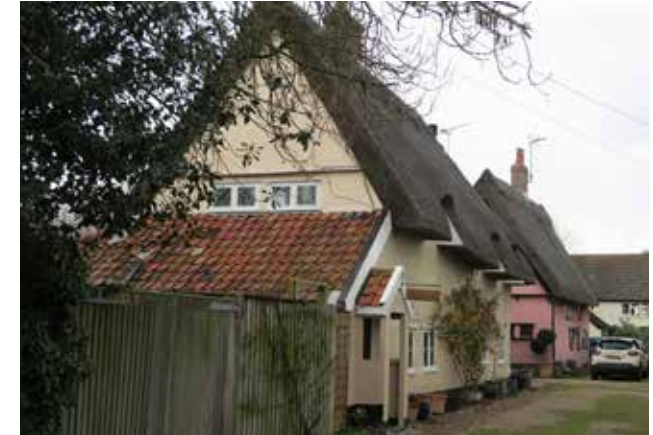
Thatch and pantile roofing.
