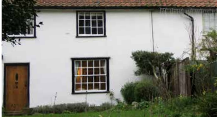
Painted front door and window trims.
