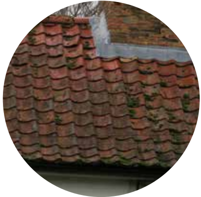
CLAY PANTILE ROOF
