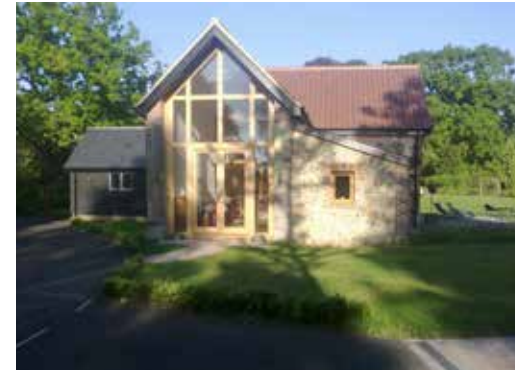
Figure 49: Barn conversion - National Federation of Builders Awards 2013, Refurbishment of the year 2012 (Top Prize); Local Authority Building Control Award 2013 (Finalist) (photo courtesy of owner)
