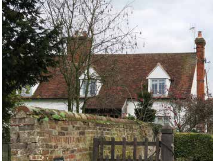
Gabled dormers on clay plain tile roof (back) and brick wall (front)
