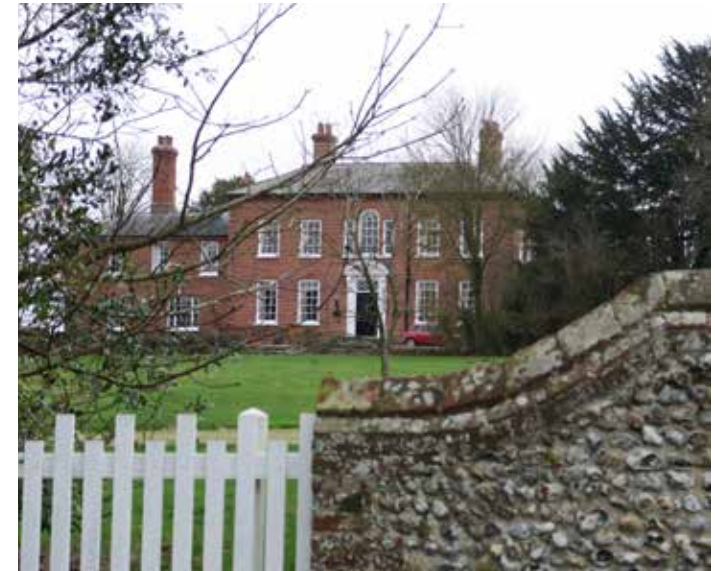
Figure 6: The 18th century Grade II* listed Old Rectory.
