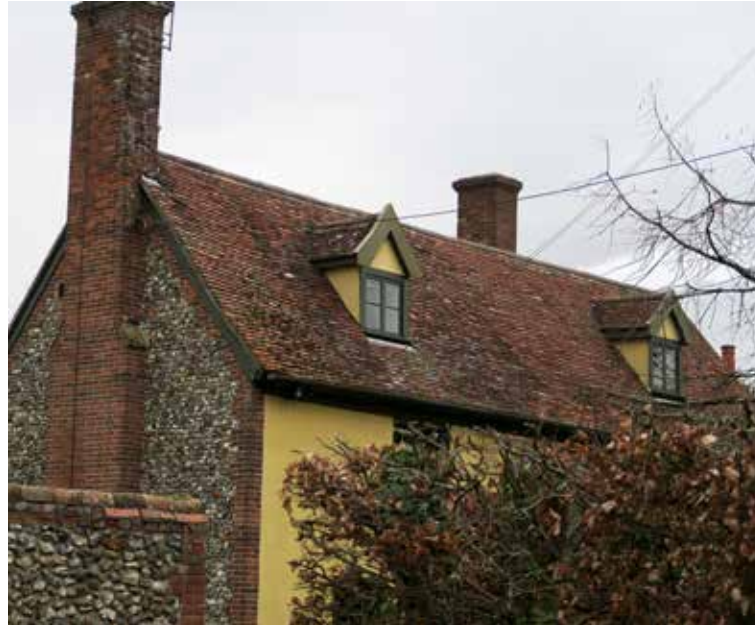
House with main façade in render and side in flint and brick.
