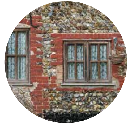
FLINT FAÇADE WITH RED BRICK WINDOW TRIM
