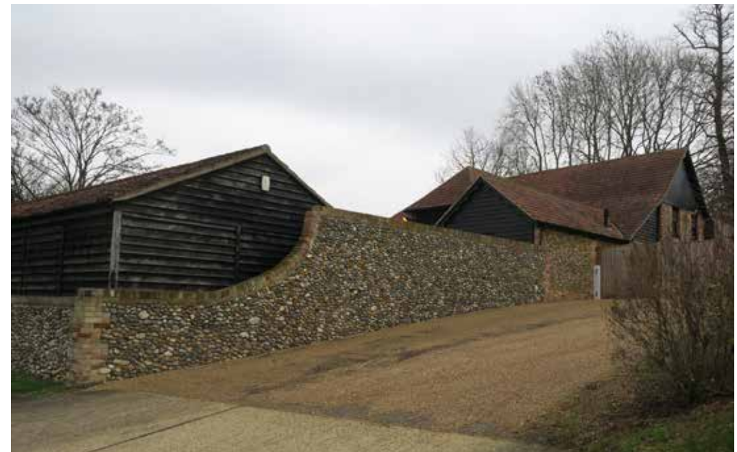
Figure 36: Pantile cottages with a diversity of roof styles, orientations, and pitches.
