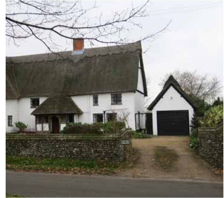
Figure 31: Low flint and brick property wall.
